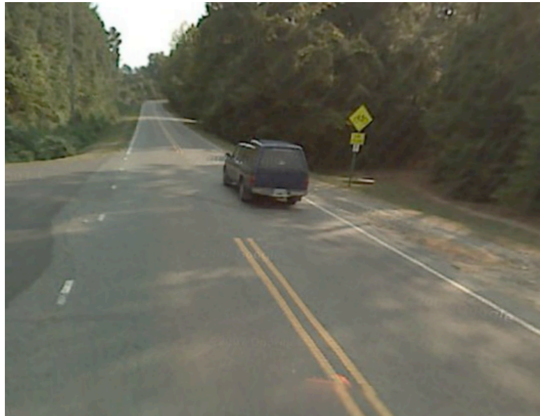
Figure 2. The sign says SHARE THE ROAD, but the lanes are not wide enough to share side-by-side within the lane. Estes Drive Ext., Carrboro, NC.
