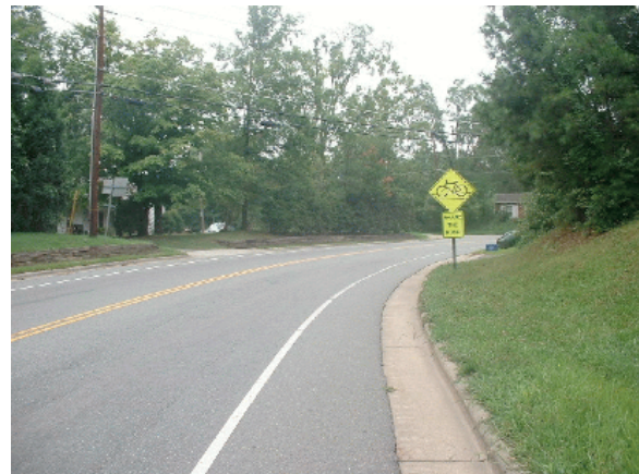
Figure 12. The SHARE THE ROAD combination sign used on a 25 mph road with a Bike Lane is a misuse of the sign. N. Greensboro St, Carrboro, NC.
