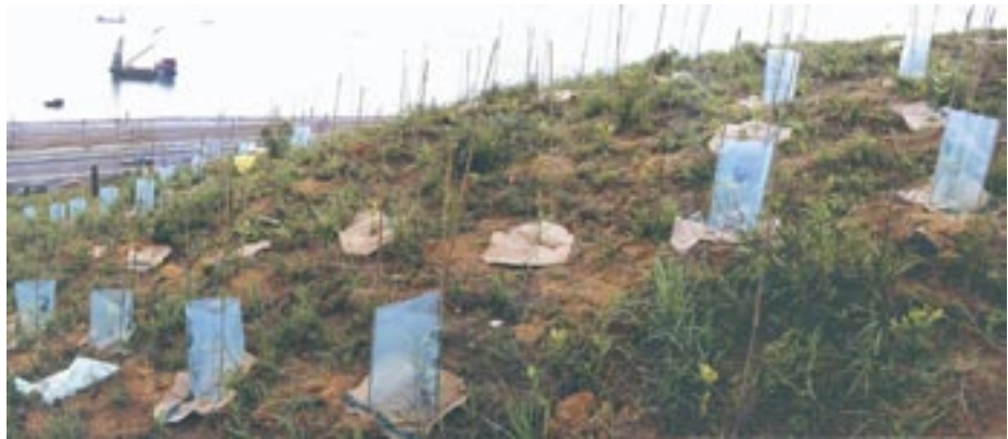
Fig 38. Tree guards set up on the exposed hill slope at Tung Chung, Lantau.
