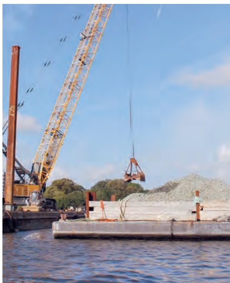
A mix of shell and stone was used to create oyster habitat in the Eastern Branch of Virginia's Elizabeth River. (Courtesy of the Virginia Marine Resources Commission)
