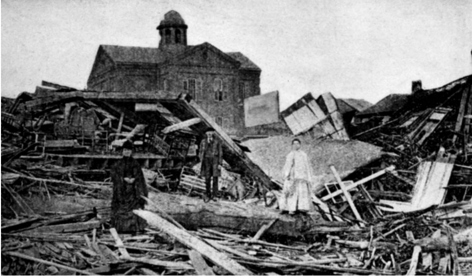
Figure 1. Damage after the Galvestone hurricane of 1900. Photo courtesy of NOAA.
