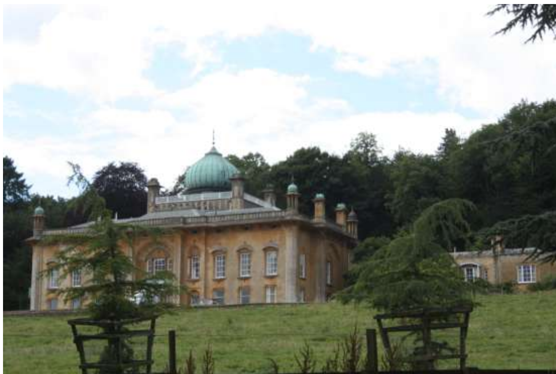
Figure 2: East façade, Sezincote; the copper Mughal-style dome dominates the skyline. Photograph by Jan Sibthorpe © 2013.
