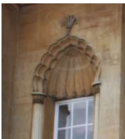
Figure 4: Detail of east façade, Sezincote, showing ‘peacock tail’ arches over the windows. Photograph by Jan Sibthorpe © 2013.
