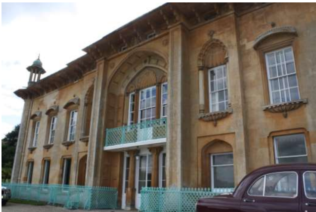
Figure 3: Detail of east façade, Sezincote, showing the chajja (deep overhanging eaves), one of four chattris (minarets) marking the corners of the central block and two-storeyed gateway style entrance. Photograph by Jan Sibthorpe © 2013.
