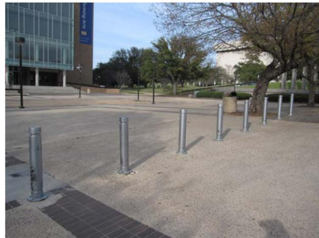
Where temporary vehicular access is required, bollards shall be removable or retractable
