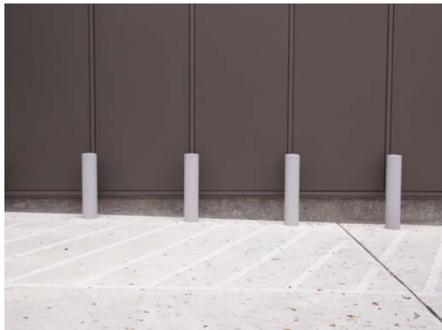
In service areas with low pedestrian use and visibility, simple pipe bollards with a powder coat paint finish of compatible color with the building are acceptable.
