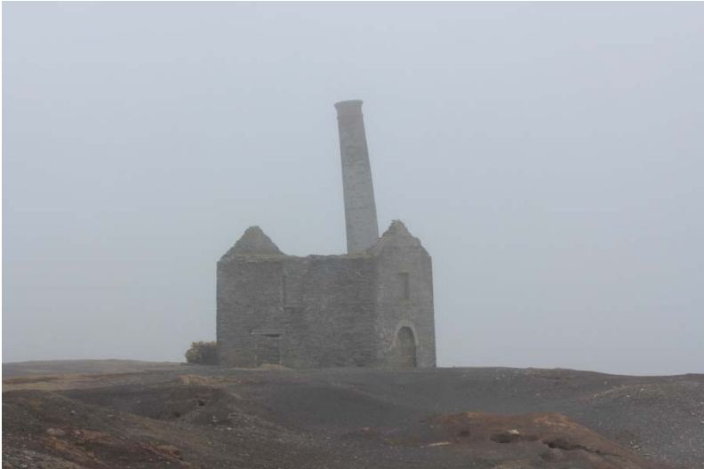
The old mine building. The chimney was like that before we arrived, honest.... Image © John Wardle
