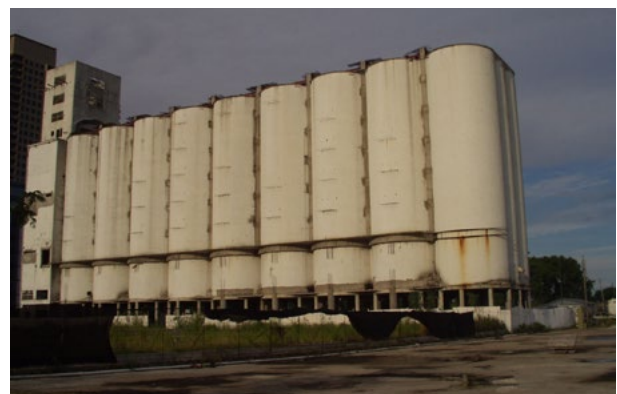
Silos of the National Grain Board.
