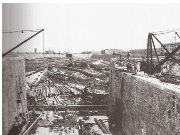
Construction works on the port. Dock 2. Rimathé, 1890.
