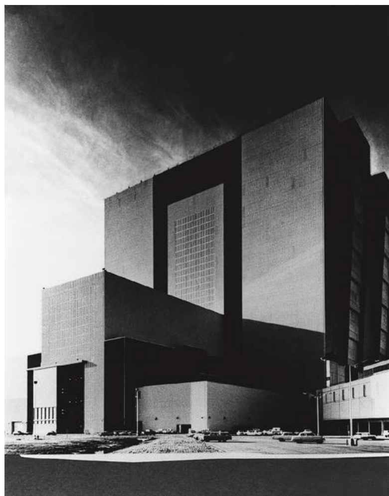
i fronti sud e est / south and east facades
