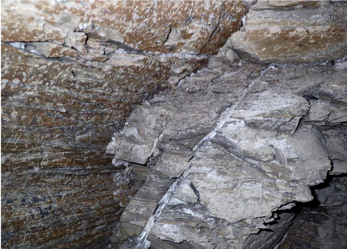
Figure 14. Shale wall (left) with gypsum-wedged shale (right). Height and width are about 1 m.
