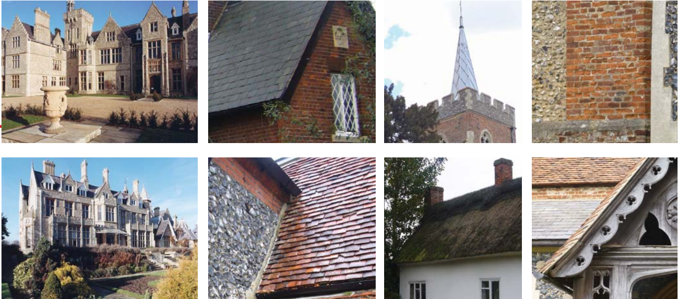
STONEMWORK OF GILSTON HOUSE. KNAPPED FLINTS, SLATES, TILES, THATCH AND WEATHERED TIMBERS OF NORTHERN AND EASTERN VILLAGES
