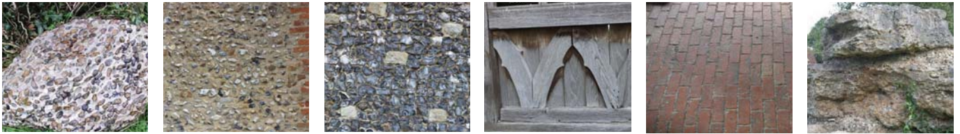
ESSEX AND HERFORDSHIRE PUDDINGSTONE, KNAPPED FLINT, WHOLE FLINTS AND WEATHERED TIMBERS
