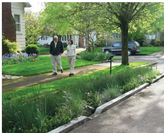
RAIN GARDEN SUDS PLANTING
