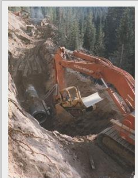
Municipal Pipeline Construction
