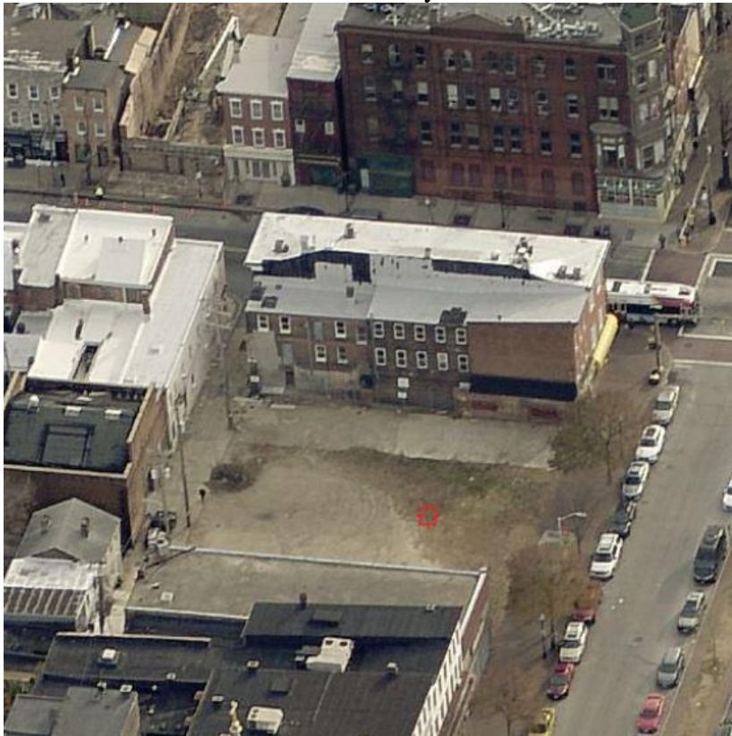
View 421 South Broadway from the north
