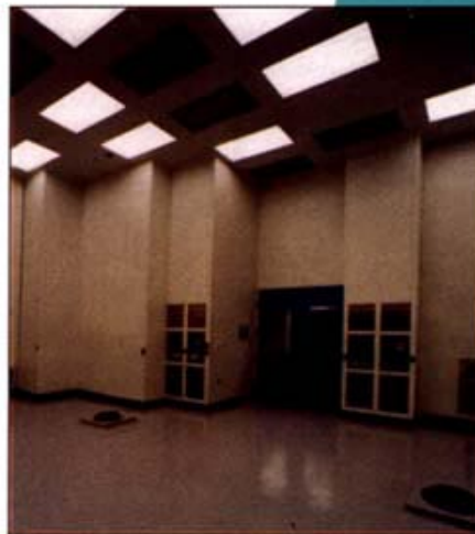
Photo 4. Modular cleanrooms present virtually unlimited opportunities for rearrangement, even dismantling and moving, of entire facilities or their parts.
