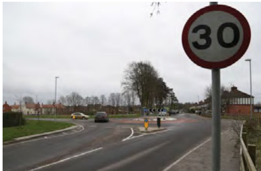
Above: Image of upgraded road network at Durrington
