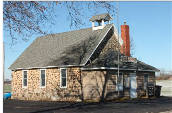
Stone School, 1869 N1409 Fremont Road, Town of Cold Spring
