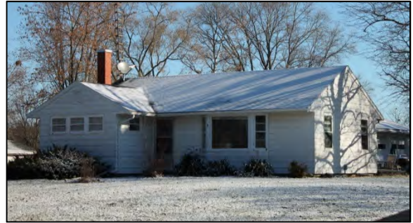
Seth Nathan House, 1950 N354 Cold Spring Road, Town of Cold Spring
