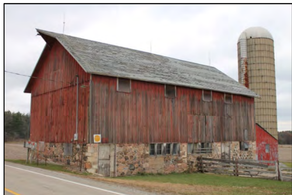
Gilbert Farmstead Barn, <1937 N2531 County Highway Z, Town of Sullivan
