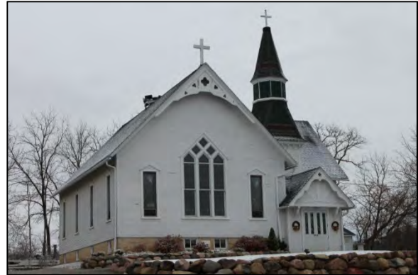
Hebron Methodist Episcopal Church, 1899 N2349 County Highway D, Town of Hebron
