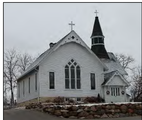
Hebron Methodist Episcopal Church, 1899 N2349 County Highway D, Town of Hebron
