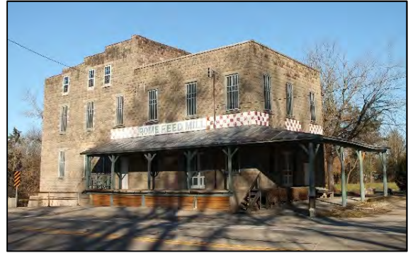
Rome Feed Mill, 1924 W1860 Main Street, Town of Sullivan
