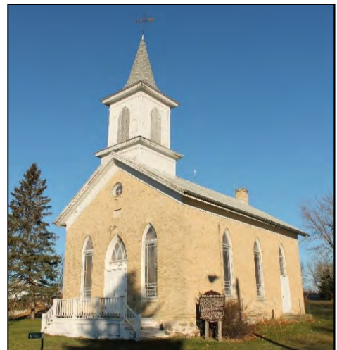
Evangelical United Brethren Church, 1868 W1984 Main Street, Town of Sullivan
