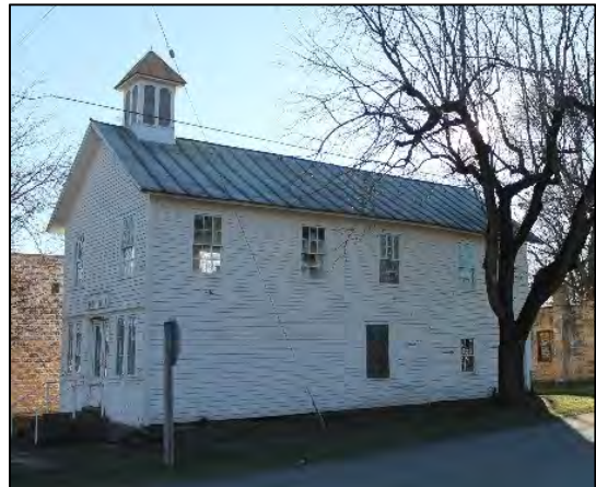
Ungermire Hotel / Old Rome Village Hall, 1879 W1935 Main Street, Town of Sullivan
