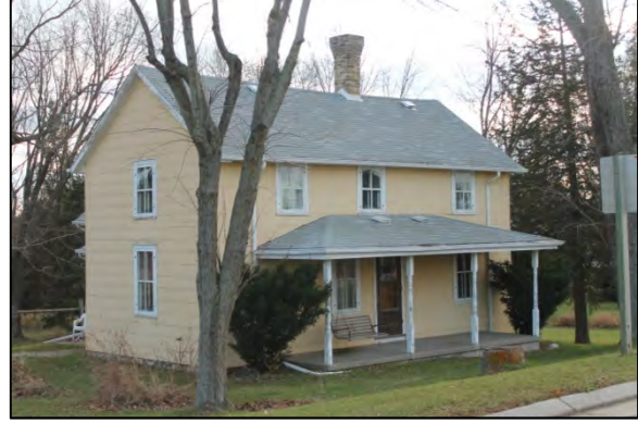
F.J. Holtz House, 1860 W857 US Highway 18, Town of Sullivan
