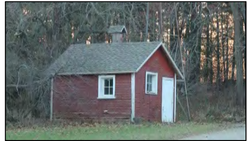
E. Uglow Farmstead Pump House, <1937 W114 Hooper Road, Town of Palmyra
