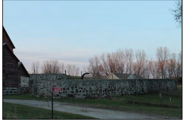
Christian Oleson Farmstead Stone Walls, <1937 N1473 Zion Road, Town of Palmyra
