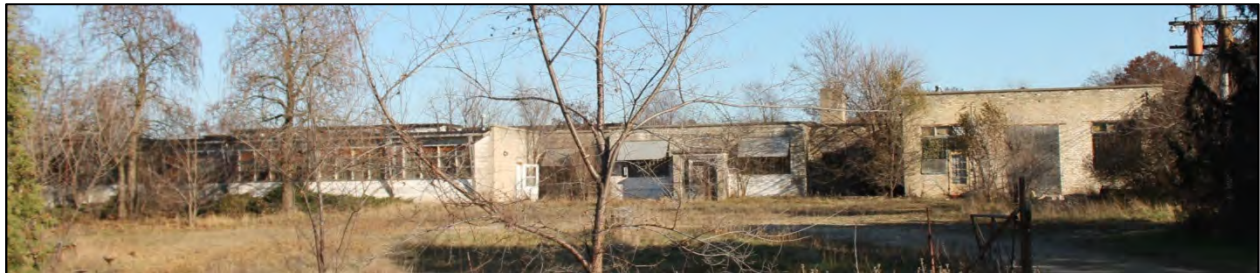
Young Engineering Company Snow Valley Plant, 1954 N252 County Highway H, Town of Palmyra
