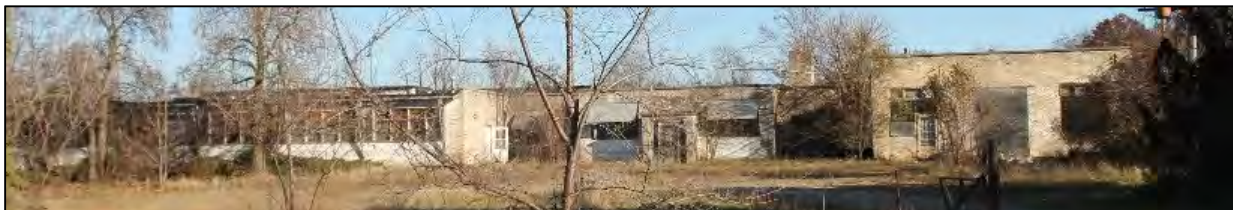
Young Engineering Company Snow Valley Plant, c.1950 N252 County Highway H, Town of Palmyra
