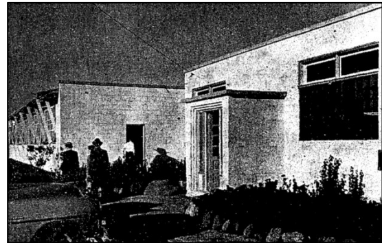
Young Engineering Company Snow Valley Plant Addition in 1954 (Janesville Daily Gazette Sept. 27, 1954)
