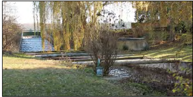
Blue Spring Lake Dam, 1927 N528 County Highway H, Town of Palmyra
