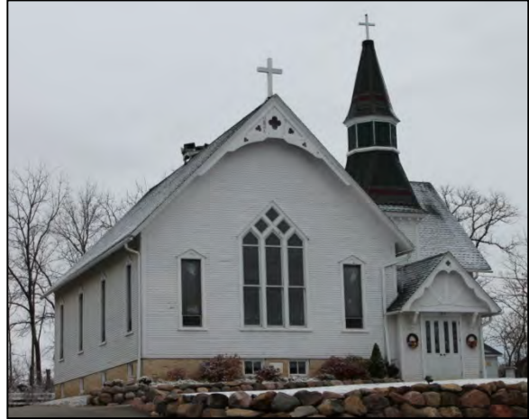
Hebron Methodist Episcopal Church, 1899 N2349 County Highway D, Town of Hebron
