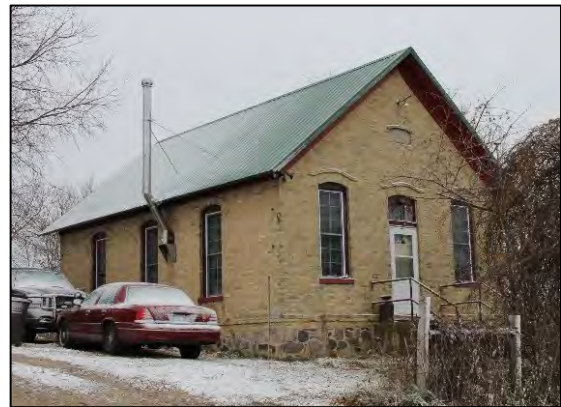
Wright’s Mill School, 1891 W3393 Hagedorn Road, Town of Hebron
