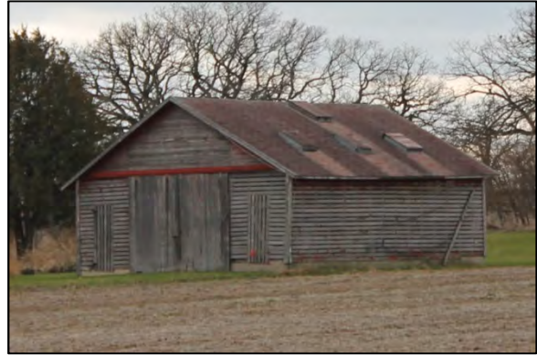
Gilbert Farmstead Corn Crib, <1937 N2531 County Highway Z, Town of Sullivan
