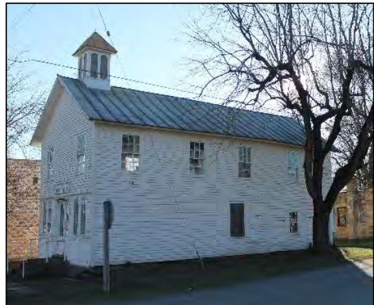
Ungermire Hotel / Old Rome Village Hall, 1879 W1935 Main Street, Town of Sullivan
