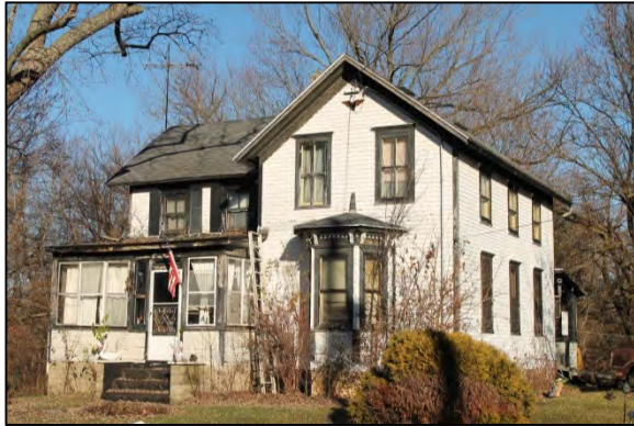
House, c.1870 W1834 Main Street, Town of Sullivan
