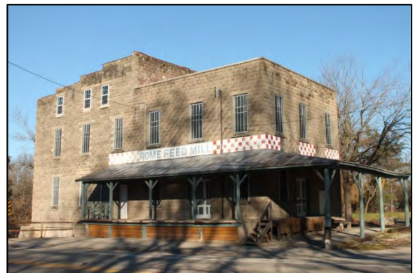
Rome Feed Mill, 1924 W1860 Main Street, Town of Sullivan
