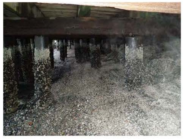
4 EXISTING TIMBER WHARF FRAMING
