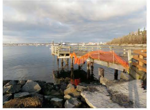
3 EXISTING TIMBER PIER (LOOKING NORTH)
