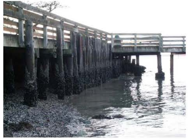
2 EXISTING TIMBER WHARF (LOOKING WEST)
