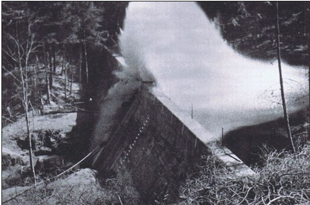
Plate 4: The Nant y Gro Dam, built to supply water for the workers’ settlement at Elan Village was breached by experiments with bouncing bombs carried out by Barnes Wallace in 1942.
