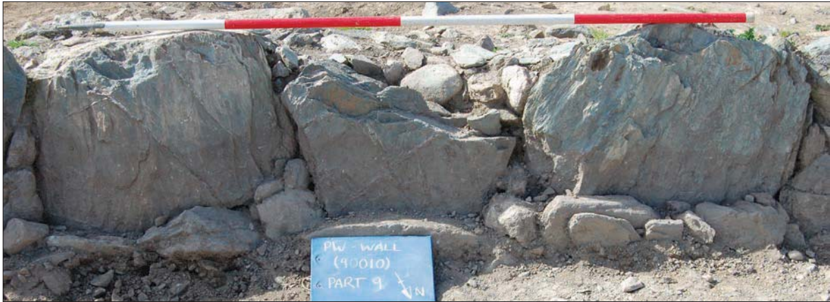
Plate 112. North-east face of wall 90010 fully exposed, showing packing stones at base
