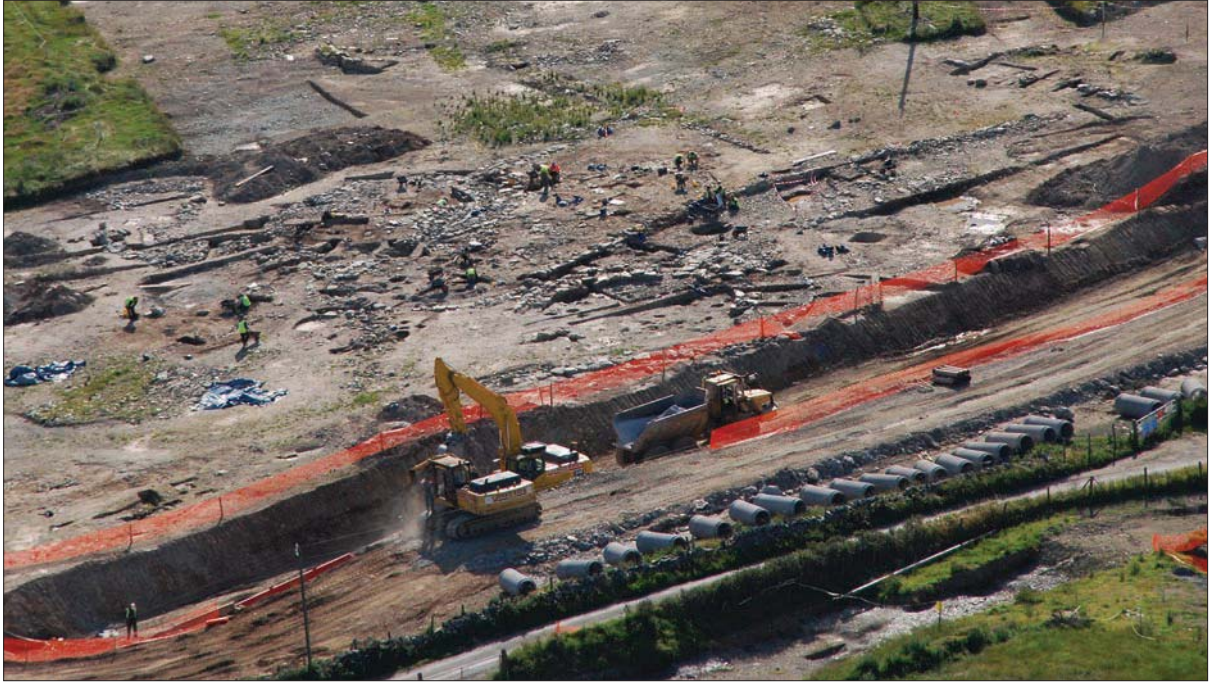
Plate 76. Conditions of excavation in Area B2 with archaeologists separated from an active haul road (photograph by David Longley)
