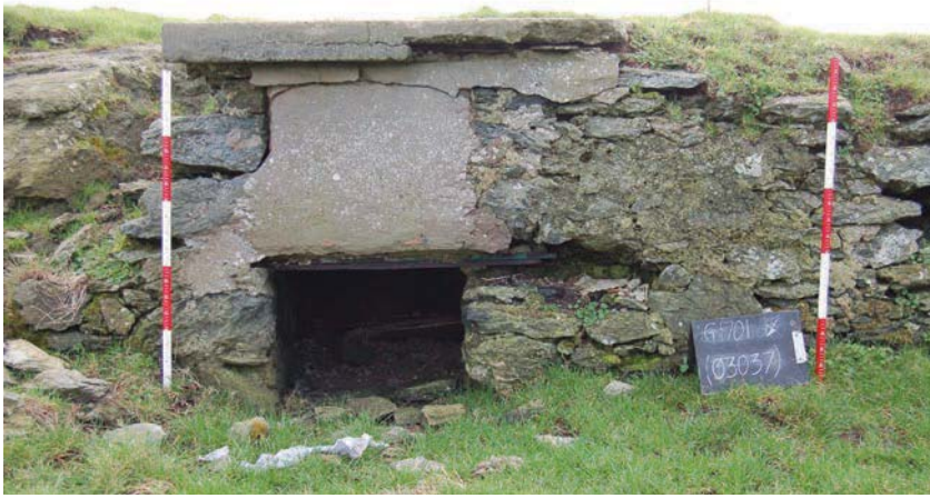
Plate 212. Small structure (03038) with concrete roof
