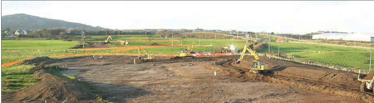
Plate 9. Machine stripping topsoil and ploughsoil
