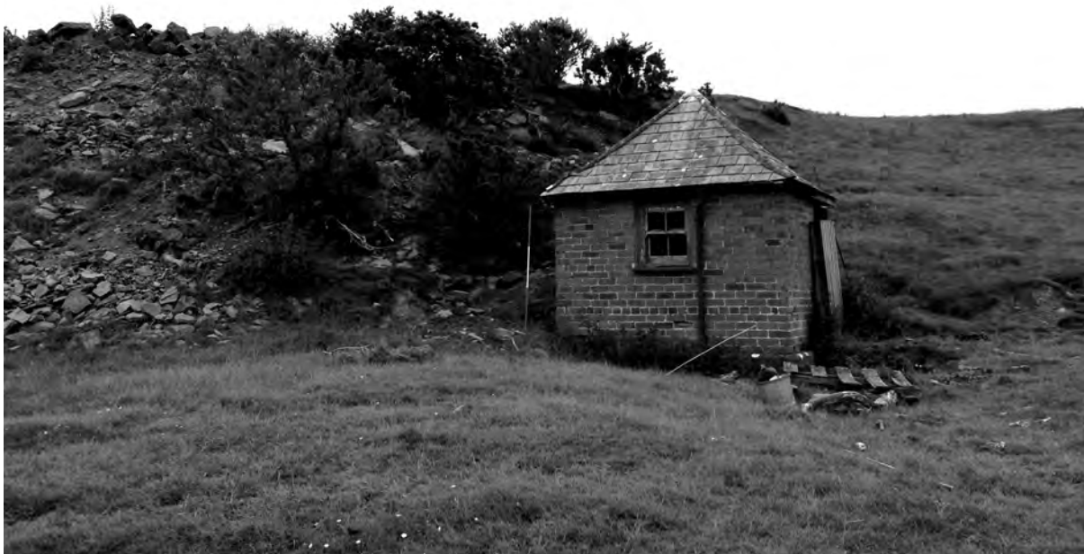
Figure 6 The pumphouse. Photo looking SE, by Dickson & Tram
