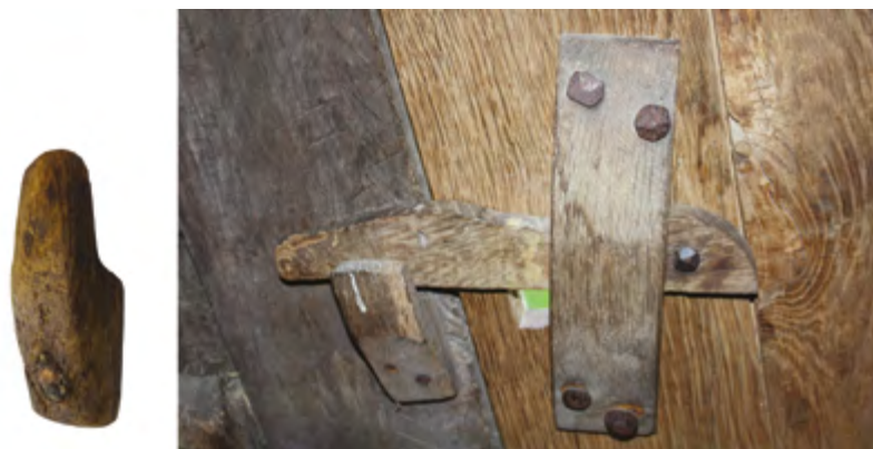
Figure 11.1 Catch from Velsen 1 (left: find number 3044, ash) and fastening mechanism with a bolt and catch on an old farmhouse door (Bokrijk Open Air Museum, Belgium) (photos: BIAX Consult).
