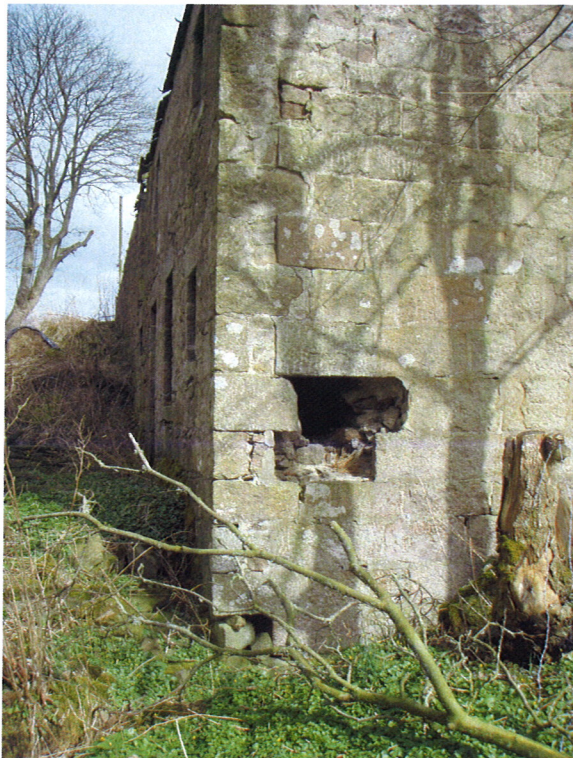
Photograph 6 – South West Corner
