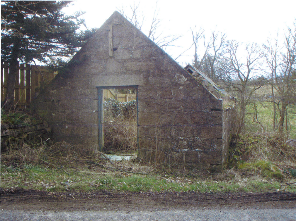
Photograph 1 – North East Elevation
