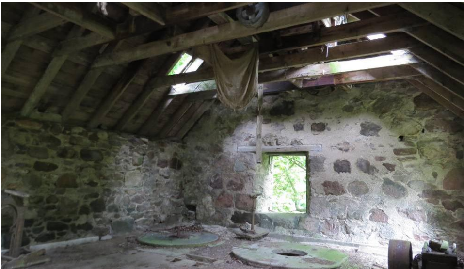
Photo 13: South gable. Roof rotten and collapsing in places. Algae on floor and walls are further evidence of damp with rainwater entering the building. There is no enclosed roof space and limited bat roost potential.
