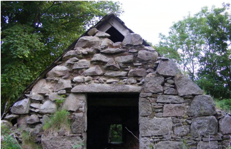
Photo 4: North elevation. Wall in poor condition, with large gap at the ridge. Large cracks are shallow and offer no bat roost potential. No evidence of bats.
