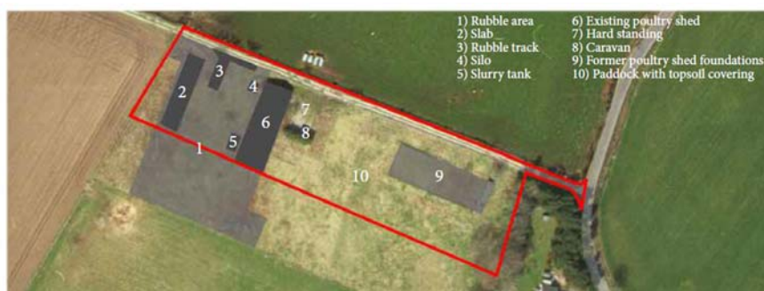
(Figure 2: Aerial View of Existing and Former Buildings/ Structures at Site)
