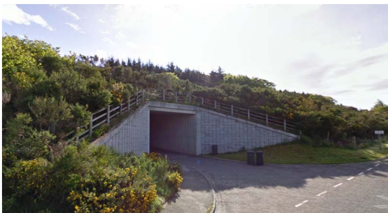
(Figure 3: Pedestrian Underpass at A96 adjacent to Bishopton)
