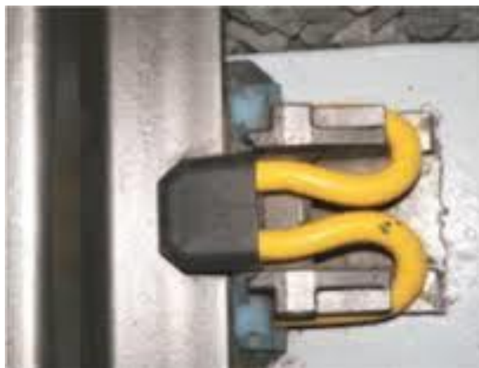
Fig. 7 - Pandrol Fastclip [10]
