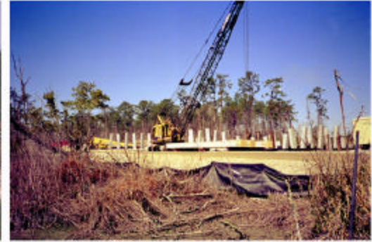
Edwards Creek Site During Construction
