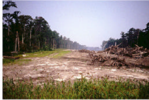
Edwards Creek Site During Clearing
