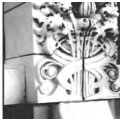
Good blending repair
