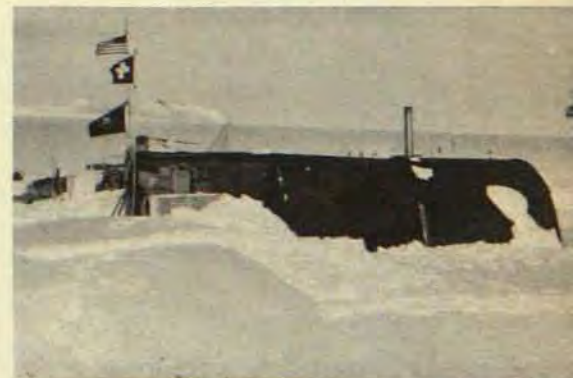
Jamesway huts, this one designed for sleeping, are the standard dwelling for Antarctic explorers.
