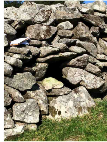
D - Chamber constructed within the wall
