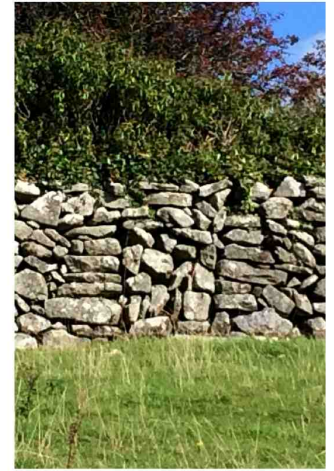
E - Junction with wall now removed
