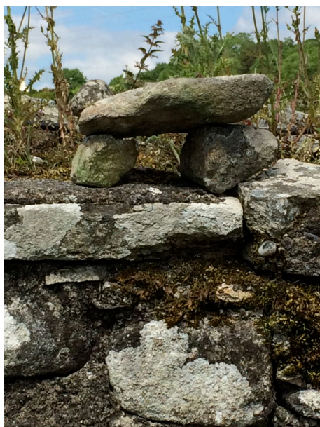
Example of a box drain built by Dranagh farmer Patrick Byrne during fieldwork
