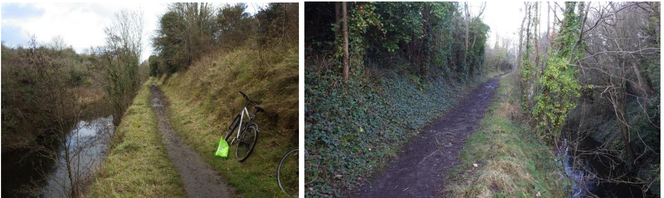
Figure 3.1: Existing towpath on the southern side of the canal between Kennan Bridge and Kirkpatrick Bridge (adjacent to the railway line)
