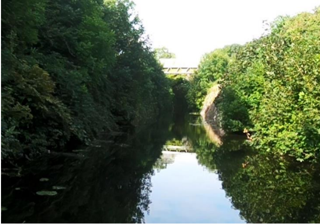
Figure 7.3 Photograph of existing southern embankment in Zone 1 (facing west toward Kirkpatrick bridge)
