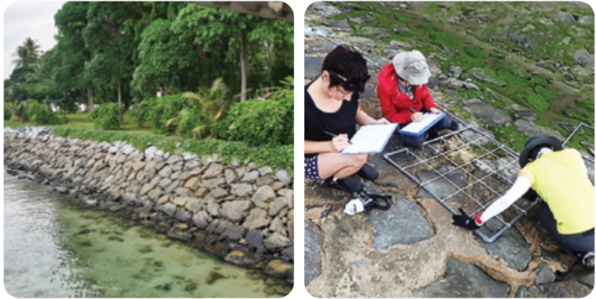
Figure 1: (a) Typical granite rip-rap seawall in Singapore (at Pulau Hantu). (b) Conducting surveys at Changi Bay.
