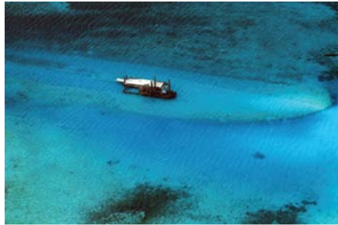
Figure 15.5 This spud barge is deepening the channel leading into the dock at Peleliu Island. It jacks itself up on legs to remain steady. There is a mechanical excavator attached to the rear of the barge; the excavator digs up the sand directly below and deposits it on the barge. The sand on the barge is taken to shore and used elsewhere. The sand removed could have been dumped alongside the barge to form a spoil bank, but if the material can be used elsewhere, it is advantageous to remove it from the site.
