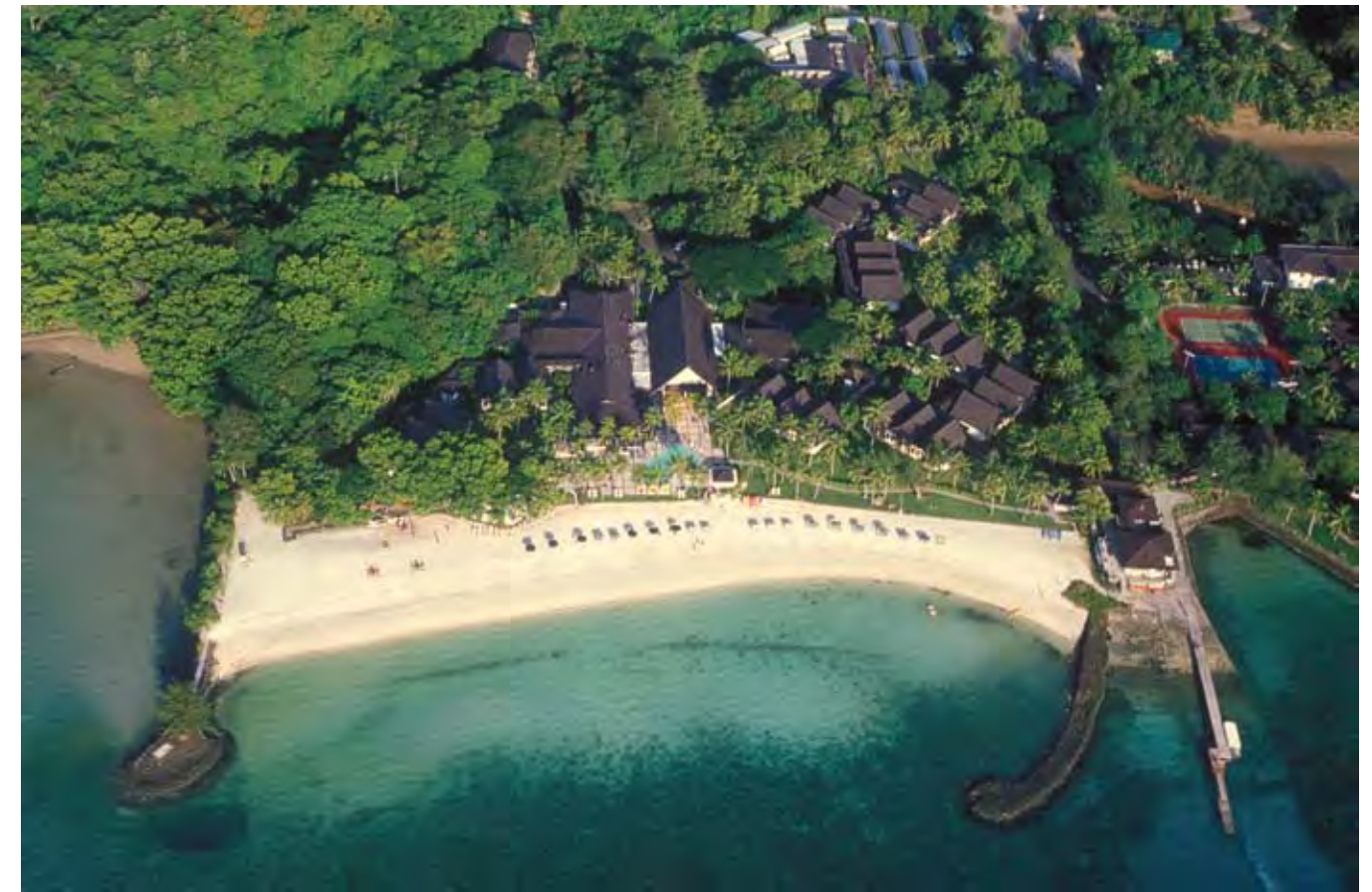
Figure 15.18 The beach at the Palau Pacific Resort is man-made. This was formerly an area of mangrove swamp shoreline, but the mangroves were removed and twin groins constructed to prevent loss of the beach sand. The beach gradually transitions to seagrass; there are small corals offshore. Visitors to the resort love snorkeling in this diverse area. They have no idea that it was once a mangrove swamp.
