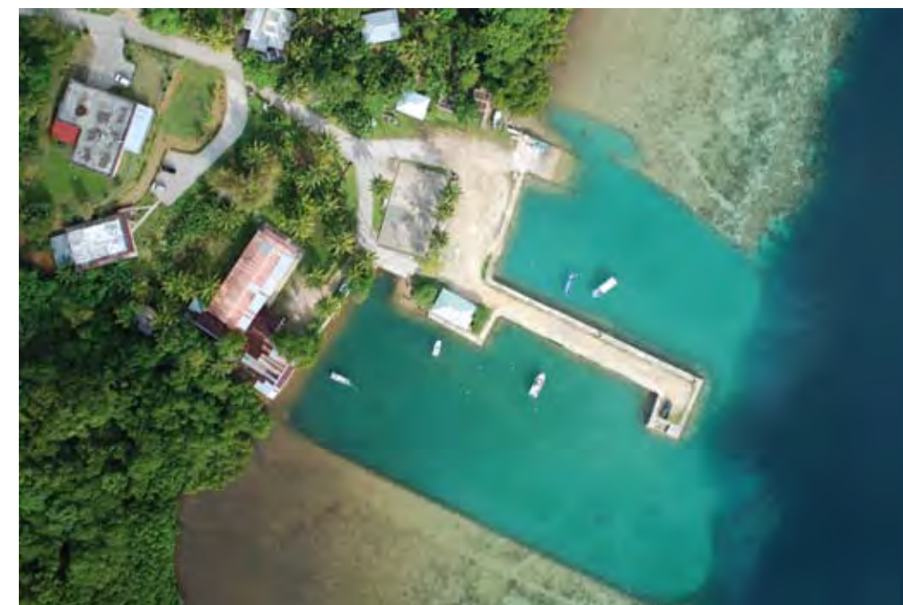
Figure 19.25 Koror and other states of Palau have seen numerous projects to develop local docks through dredging of fringing reef flats near villages. This project at Ngermid, on Koror Island, created a small boat harbor by removing shallow bottom like that seen on either side of the dredged area. Such developments are welcomed by most people, as they provide protected mooring areas and easier access to fishing grounds; boats can come and go at all tides (such flats are normally exposed at low tides). Such dredged areas also provide flat areas for public recreational facilities (basketball courts, etc.) in areas where such land is no longer available due to prior development.
