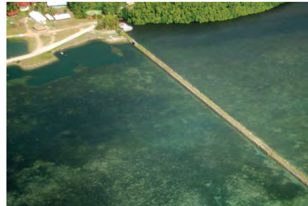
Figure 14.5 Due to the wide flats along the shore of Babeldaob, most villages need jetties that reach out into water deep enough for small boats at all tides. The jetty at in Ngechesar village in Ngechesar State is nearly 500 m long; there is a small house at its outer end. Recent dredging along the shore now allows boats to be anchored there at low tides, but access to the inner mooring area is still limited at low tide.
