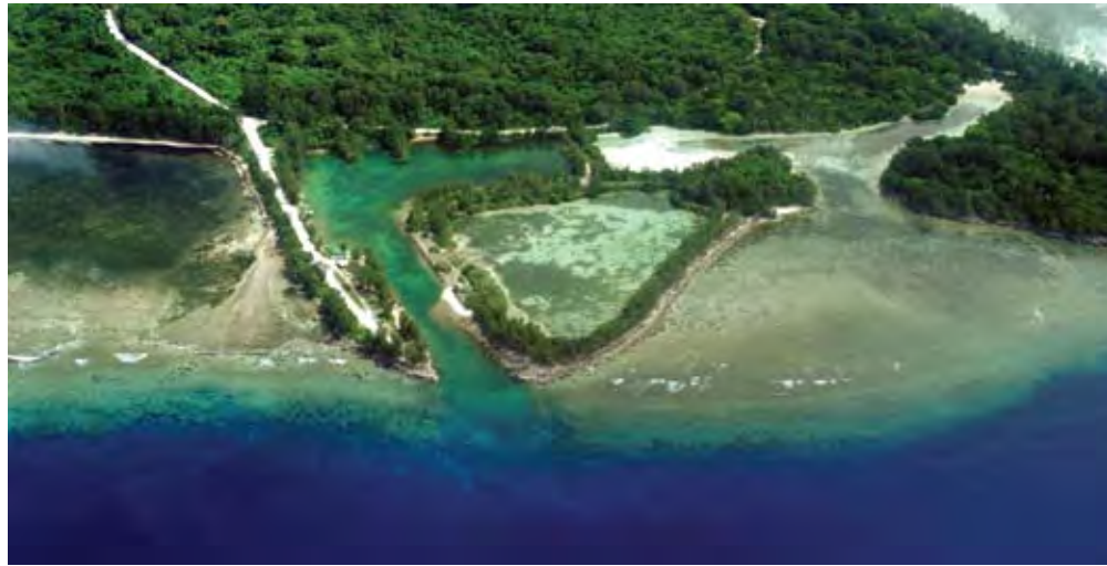
Figure 2.62 This man-made harbor at the southern end of Peleliu was built after the capture of Peleliu by US forces in WWII. A channel was dredged through the reef flat with an inner harbor area. The fill from the dredging was used to build berms that protect the harbor. Much of the inner area of this small harbor is lined with old rusty floating dock sections. The narrow insular shelf of Peleliu drops steeply at the seaward edge of the reef flat to ocean depths.
