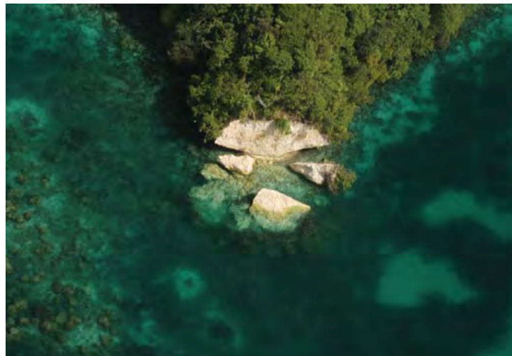
Figure 9.14 If the sea level notch around the Rock Islands is eroded too far into the island, the weight of the overhanging rock can cause the rock above to collapse. This collapse occurred in July 2005; it dropped a large block of limestone into shallow water at the corner of an island. The white limestone will gradually start being weathered and eroded by exposure to the elements and the marine communities which grow on rocky intertidal surfaces will soon add their own hues to the rock base.
