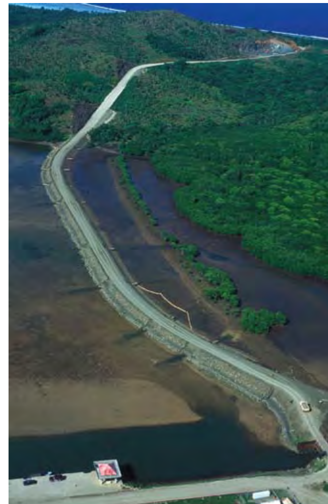
Figure 16.28 The Urung causeway is part of the Palau Compact Road. It crosses a shallow area on the west side of Babeldaob. Its placement was dictated by engineering considerations. Mangroves are growing landwards of the causeway, thanks to the many open culverts under the causeway. The culverts allow the tides to pass under the causeway into the mangroves along the island shore. Given that there was already a Japanese-era fill causeway across the area, the new causeway seems to have had little effect on the mangroves.
