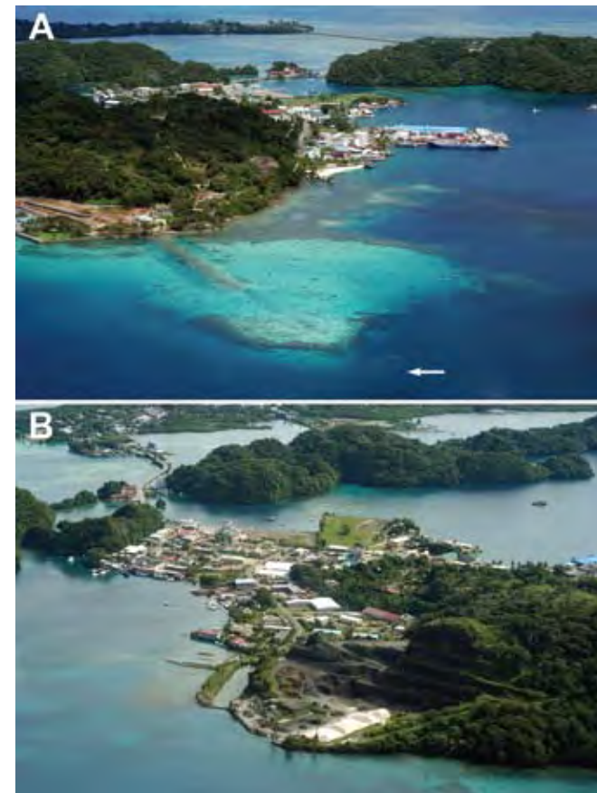
Figure 13.11 (A) The end of the outfall pipe of the Malakal Sewage Treatment plant is shown by the white arrow (lower center). The Sewage Treatment plant is located onshore and, at the time this photograph was taken, was being converted from traditional treatment to a ponding system (see Fig. 13.12). (B) The Malakal Island quarry is in the heart of the industrial area of Palau, which includes a large electrical generating plant, many workshops, boat maintenance facilities, fishing docks, and other marine-related businesses. Despite all this industrial activity, there are relatively healthy coral reef environments in this area. The high rates of flushing from tides probably protect the reefs. White coral sand obtained by sand mining on Lighthouse Reef can be seen in area of the basalt quarry. The sand is stored here after it is mined, then distributed for many purposes.
