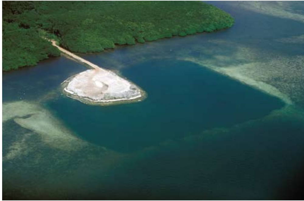
Figure 16.25 This dredging at Ngchesechang, in Ngchesar State, was done to obtain fill for road construction projects. There is now no active dredging in the area, but activities could recommence in the future.
