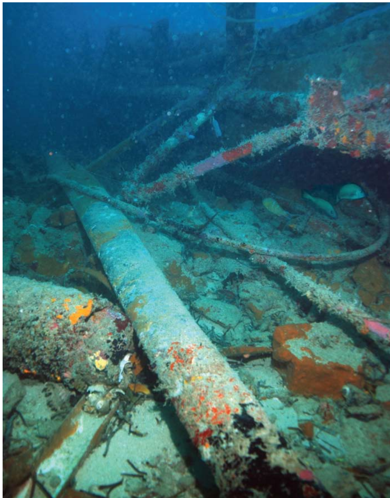
The collapse of the KB Bridge on 26 September 1996 was a disaster for Palau. This tragedy also created an immense artificial reef spanning the 300 m wide, 35 m deep channel. On portions of the sunken bridge the roadway is still relatively intact, and this view has the roadway near the top of the photograph with guard rail posts still sticking up. The box-like concrete structure of the bridge was hollow and created a large amount of cavern-like habitat that many large reef fishes prefer, hence large numbers of snappers and groupers are found on the bridge.
