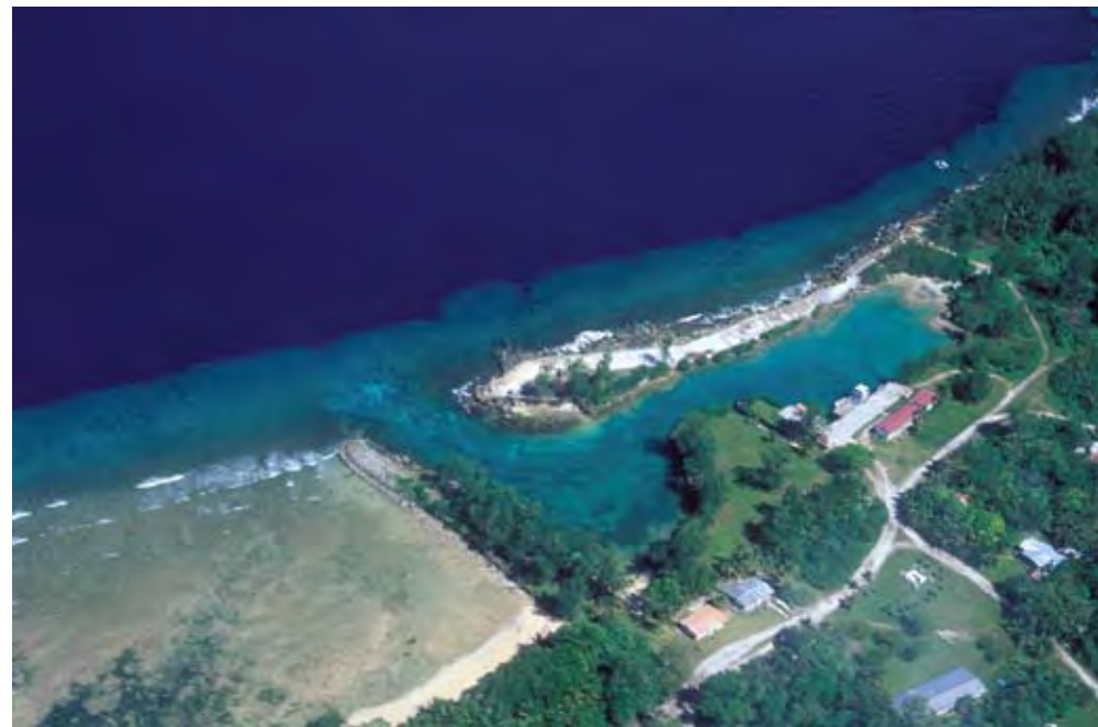
Figure 4.17 Angaur Harbor sits on the west side of the island, extremely close to the drop-off into the deep ocean. It is therefore very exposed to any swell or waves coming from the west. It is largely man-made, though it starts from a small natural harbor on the shore. The reef here has a near vertical drop off, with an extensive development of caverns and crevices on its face. The internal harbor area supports a number of coral species. Coral diversity increases towards the mouth of the harbor.
