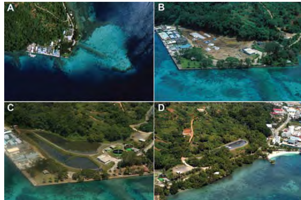
Figure 16.41 The Malakal Island sewage treatment plant has been the subject of great controversy since its construction. (A) The sewage treatment plant on Malakal Island in Koror discharges its effluent at the end of a long pipe at a depth of 15 m. The route of the pipe from shore can be seen on the right hand side of this photograph. (B) A new wastewater treatment park using a ponding system, seen under construction here. The ponds clean up sewage water, which will be discharged at the same point as the old outfall. (C) The treatment ponds after completion. (D) The header settling pond is higher than the treatment ponds. Sewage is pumped into this upper pond, where it is aerated, and flows by gravity to the lower ponds, where it slowly moves through the system, until the wastewater is finally discharged.
