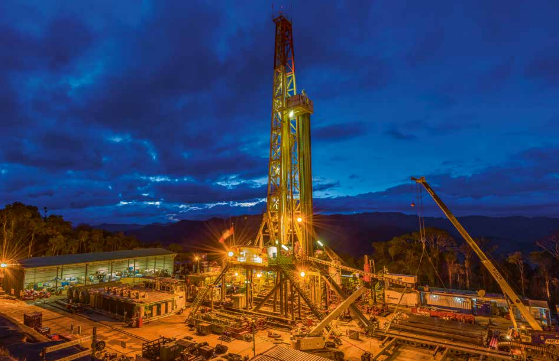
▲ Night view of the gas exploratory platform in Amarakaeri | Vista nocturna de la plataforma exploratoria de gas en Amarakaeri
