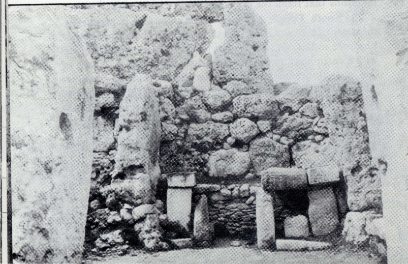
18. Ġgantija: Rear niche and back wall of North Temple
