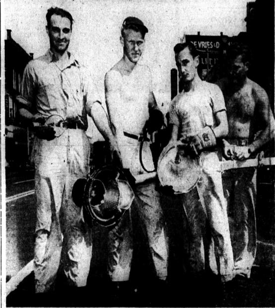
A crew erecting new boulevard lights on Eighth St., pauses to show a Sentinel photographer some of the parts that go into a modern street light. On the left is Harold Johnson, foreman, who displays a 620-watt bulb; in front of Max Davenport is a reflector assembly designed to put maximum light on the street. Harry Draime displays the glass bowl cover and Hack Watson the supporting bracket. A Three Rivers company holds a contract
