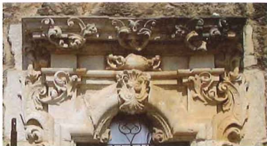
Fig. 8. Detail of the Sacristy Window during cleaning (left) with the Sensi-Clean microabrasive cleaning system.
