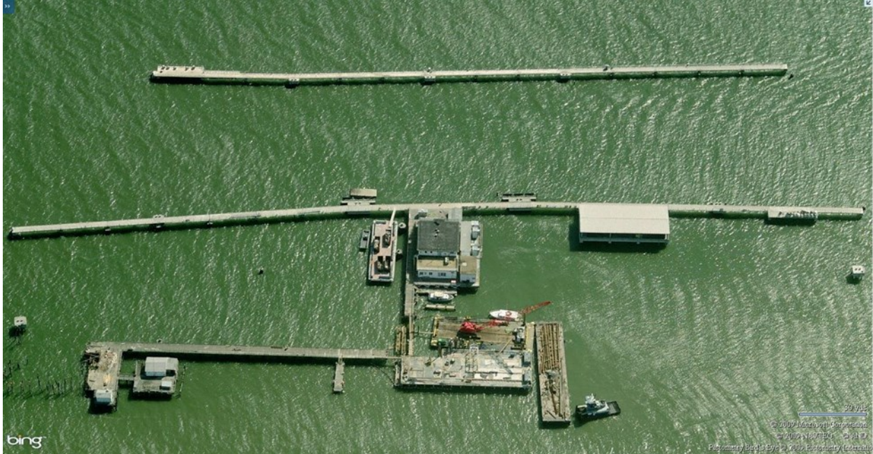
Figure 2: Magnetic treatment facility at Norfolk.
