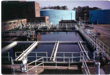
A rectangular settling tank
