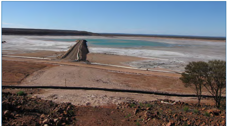
Plate 3. Overview of TSF cell 3, May 2006.
