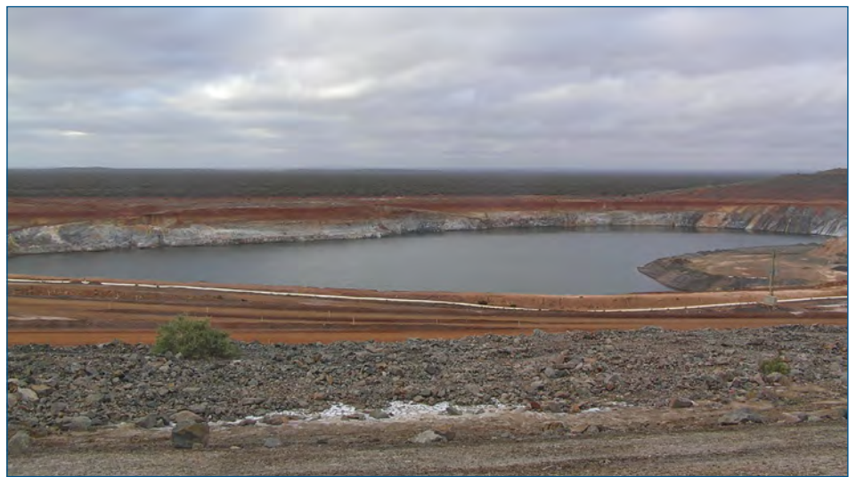
Plate 32. Winditch Pit taken from the TSF cell 2 wall.
