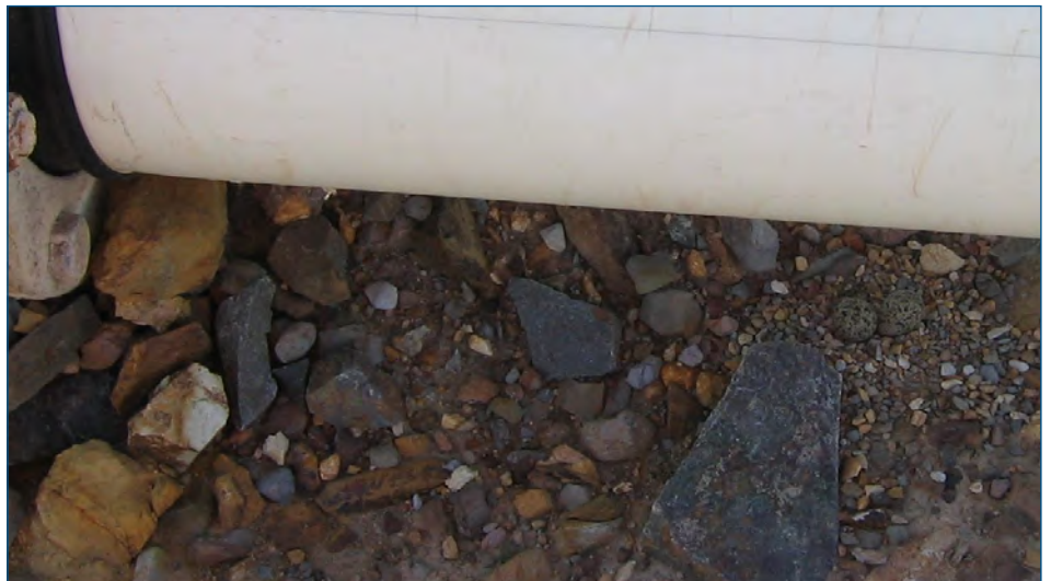
Plate 20. Location of Red-capped Plover nest next to tailings pipe on the decant finger.
