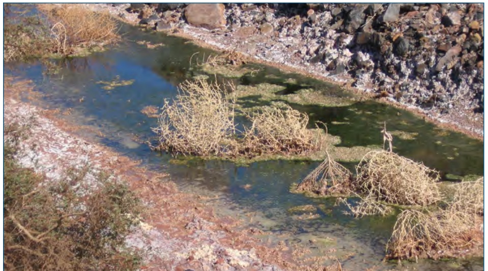
Plate 29. The seepage trench showing pooling, vegetative debris and algae.
