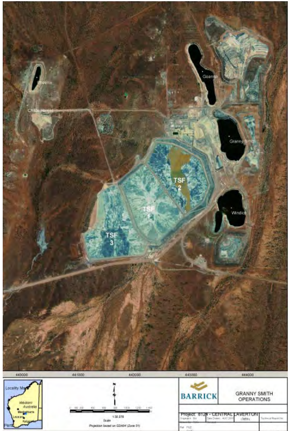
Figure 1. Aerial photograph of the mine site (August 2010) showing TSF cells and adjacent pits
