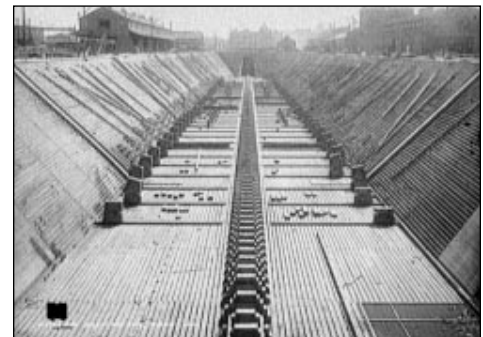
Figure 86: The Great Dry Dock, Newport News, Virginia, ca. 1905. (Photograph from the Detroit Publishing Company courtesy of the Library of Congress)
