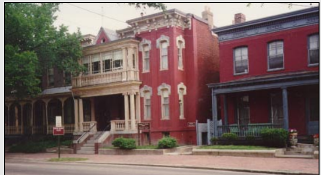
Figure 92: Maggie L. Walker Streetscape, Jackson Ward, Richmond, Virginia. (Photograph courtesy of the National Park Service)
