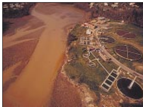
Figure 114: Water Filtration Plant, Occoquan, Virginia, 1973.
