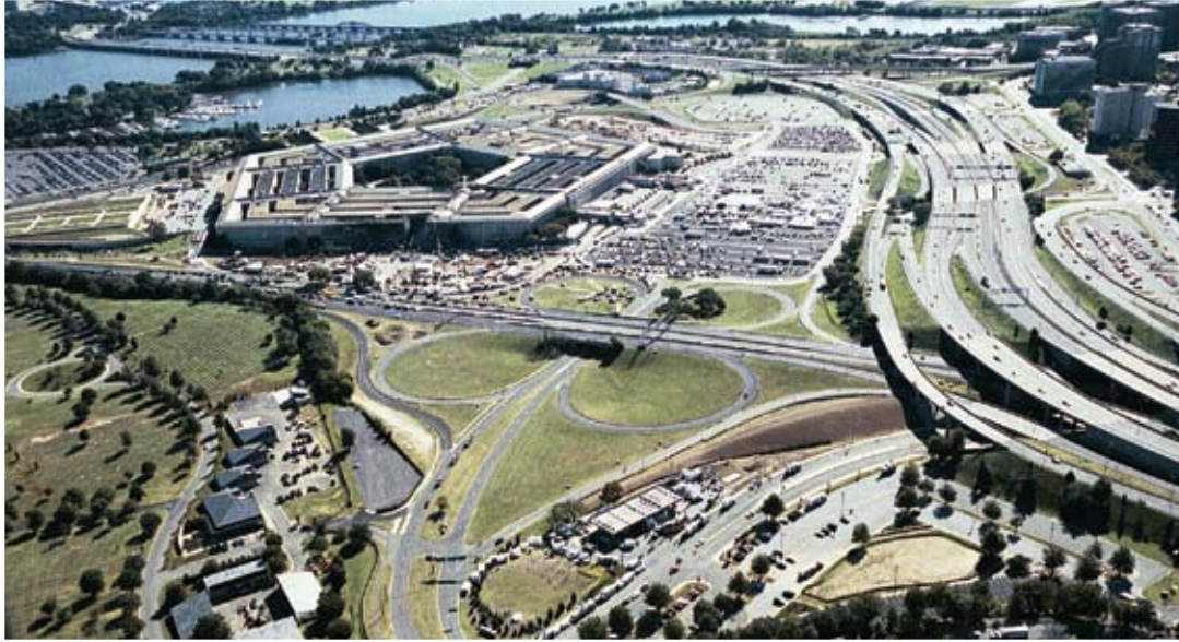
The tremendous size of the Pentagon complex can be seen in this photo, which shows nearby highways and bridges.
