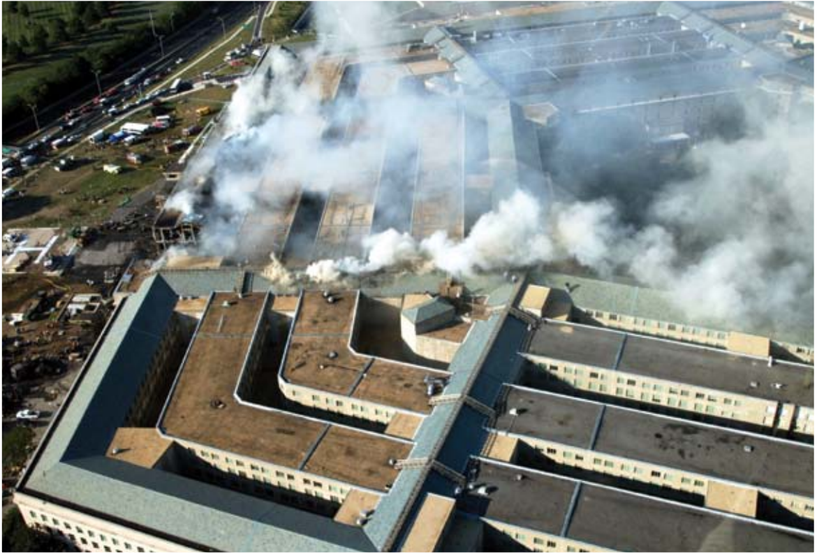
Early in the incident, fire was blowing out of the third ring of the structure.
