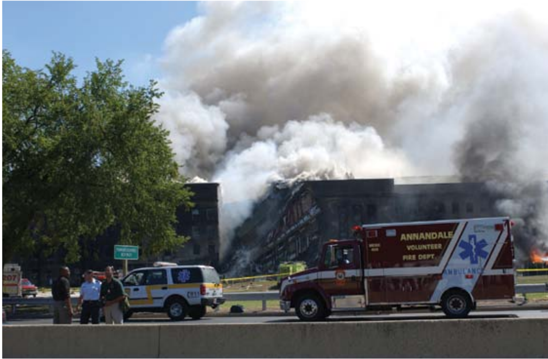
EMS vehicles were staged adjacent to the triage and treatment areas, with convenient access to the nearby highways.
