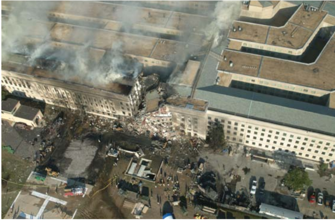
The wedge where the aircraft impacted had just been remodeled and hardened. Impact anywhere else would probably have caused more damage and fire extension.
