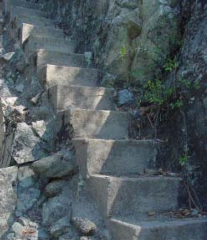
* The suspension bridge steps
