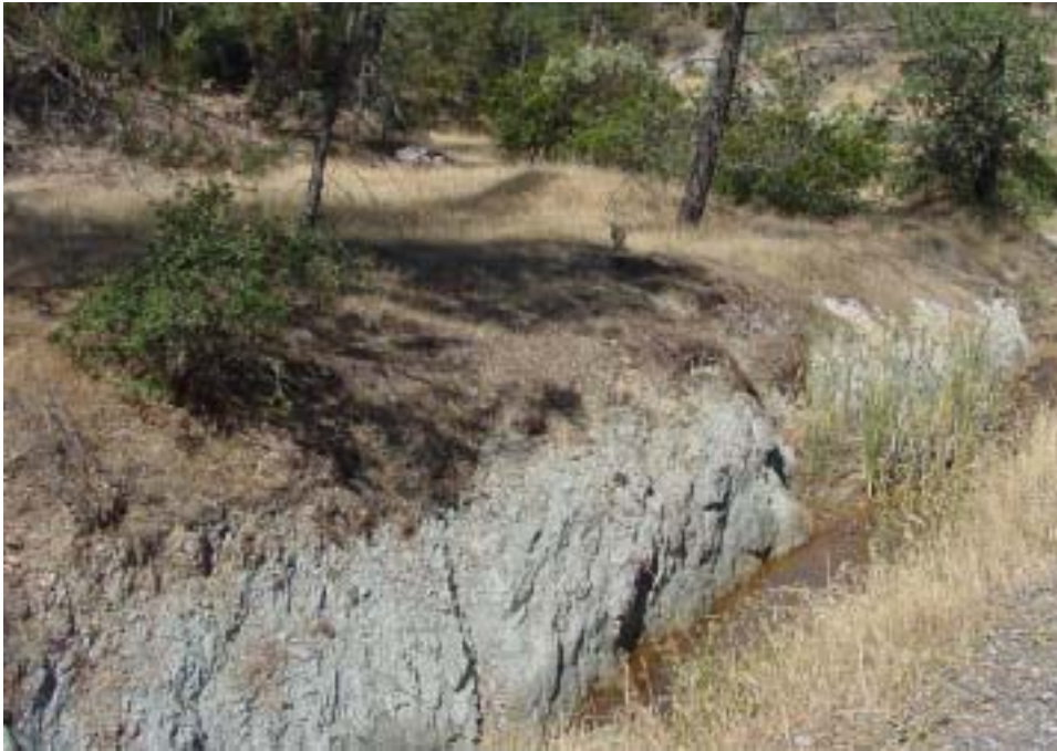
* Hoadley Fault area
