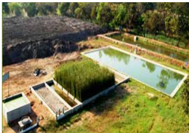
Constructed wetland facility developed at KCP Sugar Industries to treat effluent from distillery
