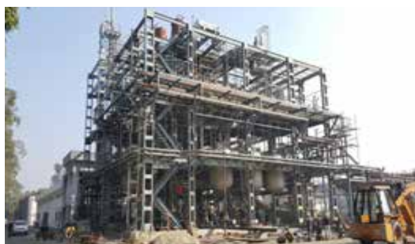
DBT-ICT Centre 2G Ethanol Technology & pilot plant at (10 Tons biomass/day) IGL Kashipur
