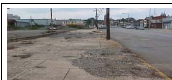
Plum Street @ 3 rd St. Sidewalk Improvements
