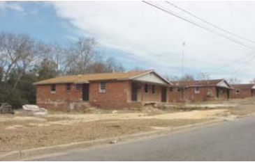
Abandoned Housing Complex
