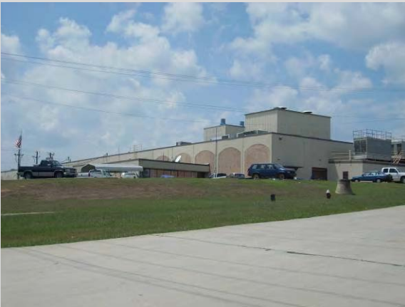
Much of the industrial development along SR4 47 is concealed from the highway.
