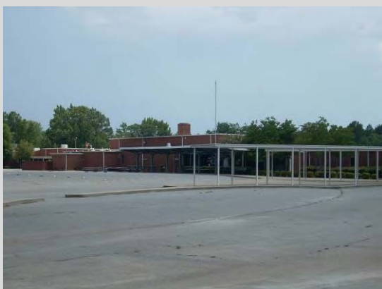
The soon to be abandoned Washington-Wilkes middle/high school is located in close proximity to Wills Memorial Hospital. The school board owned property contains multiple acres – and multiple redevelopment opportunities for the community.
