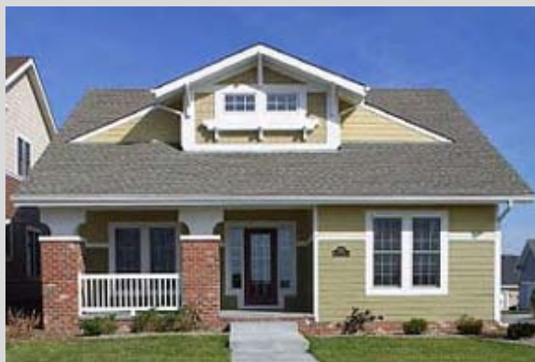
Within revitalization residential areas, emphasis should be placed on incorporating design features – such as front porches and rear garage access – that are complimentary to existing historic areas.
