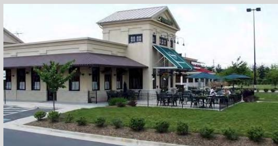
Even on major thoroughfares, new commercial development can be designed to incorporate pleasant outdoor gathering areas, landscaping, and quality building features and materials.
