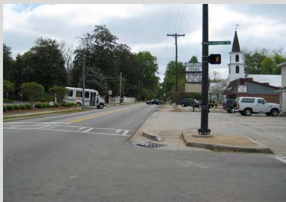
Neighborhood thoroughfares in Washington are often unfriendly to pedestrian activity or aesthetically unpleasing. This segment of E. Robert Toombs Avenue has wide travel lanes, no on-street parking, wide expanses of paved areas and few design requirements.
