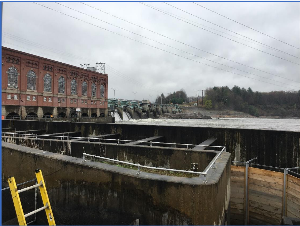
Vernon Dam and Fish Ladder
