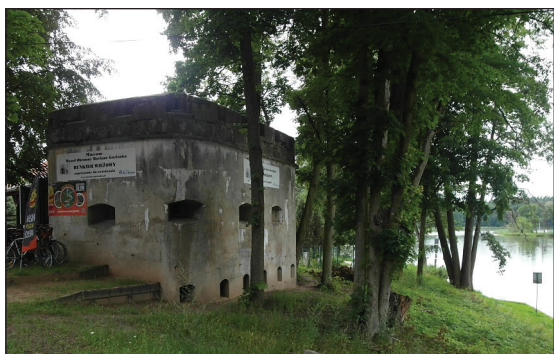
Plate VI. Guzianka, bunker by the lock (Photograph I. Lewandowska 2020).
