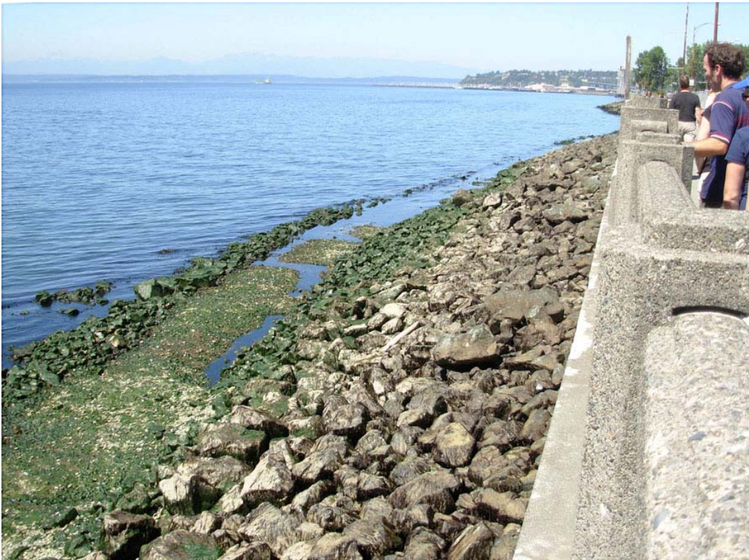
The habitat bench after construction at low tide.
