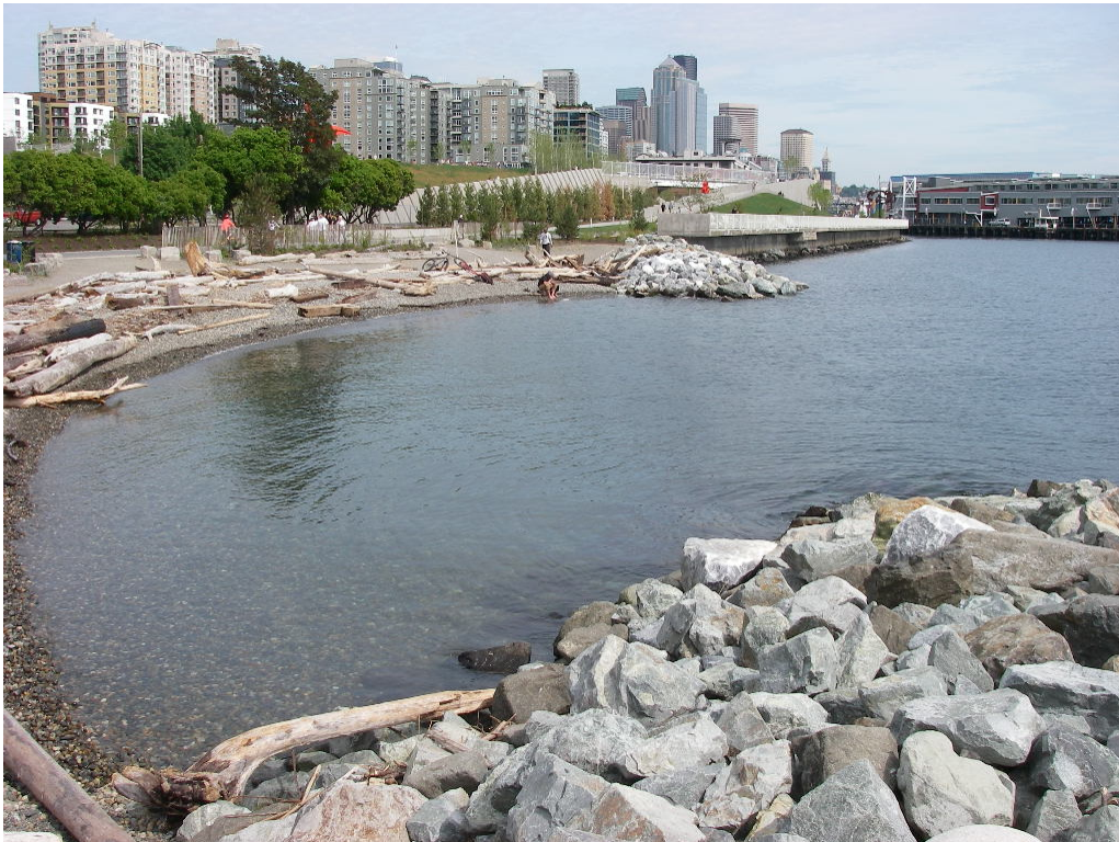
Figure 1. OSP after construction at high tide, showing inundated pocket beach and habitat bench.
