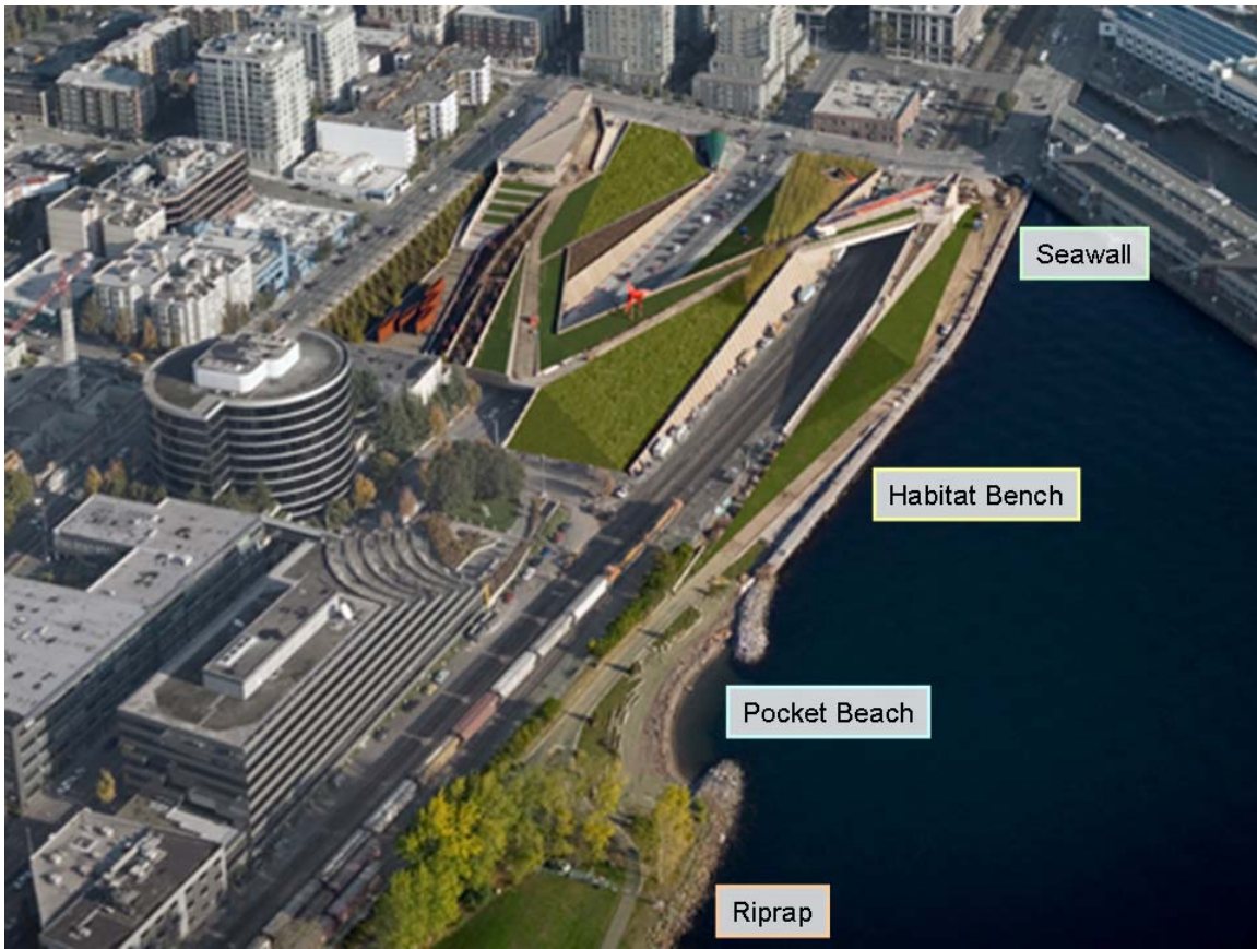
Figure 2. Aerial view of the Olympic Sculpture Park site after construction, showing general sampling locations.
