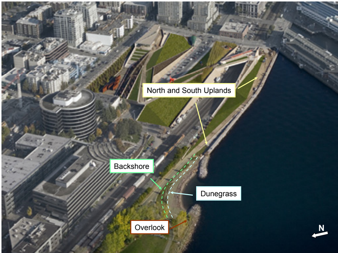
Figure 6. Aerial view of the Olympic Sculpture Park site after construction, showing vegetation sampling locations.
