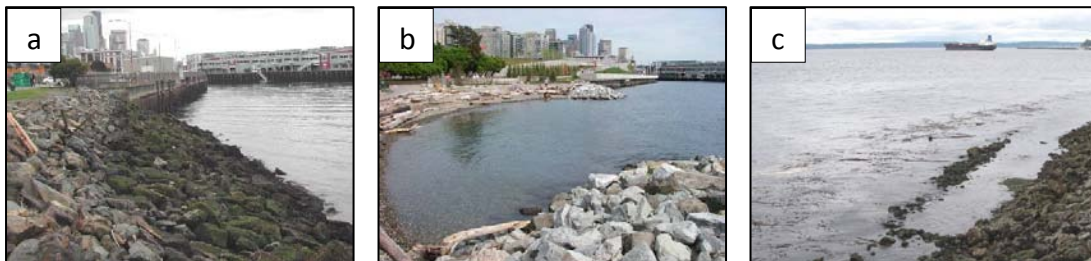
Figure 2. Photographs of the Olympic Sculpture Park (a) pre-enhancement riprap and seawall armoring, (b) post-enhancement pocket beach at high tide (habitat bench is under water) and (c) habitat bench at low tide showing kelp on the outer margin. The pocket beach replaced riprap armoring, and the habitat bench enhanced the existing seawall. Dunegrass and riparian vegetation were planted around the pocket beach, and a ‘vegetation swath’ was planted in the uplands above the habitat bench. Riprap seen in the foreground of the pocket beach in (b) and the seawall in the background of the habitat bench in (b) were sampled as reference armored sites.
