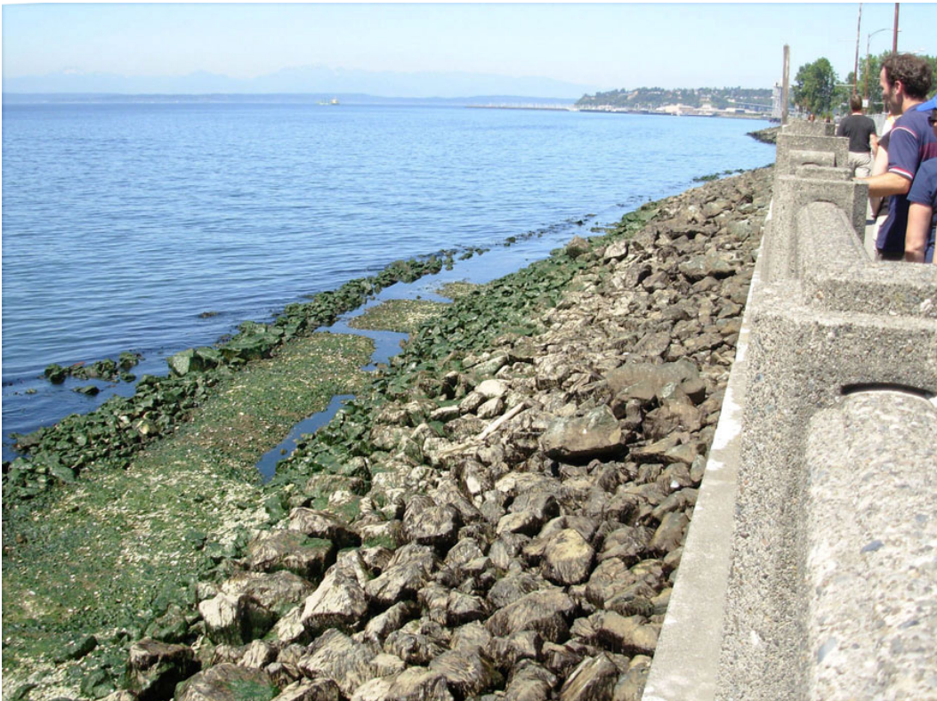
Figure 3. Photograph of the habitat bench after construction at low tide.
