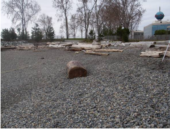
Figure 20a. Driftwood aids in retaining sediment on the berm, but logs loose on the beach can focus wave energy causing local scour.
