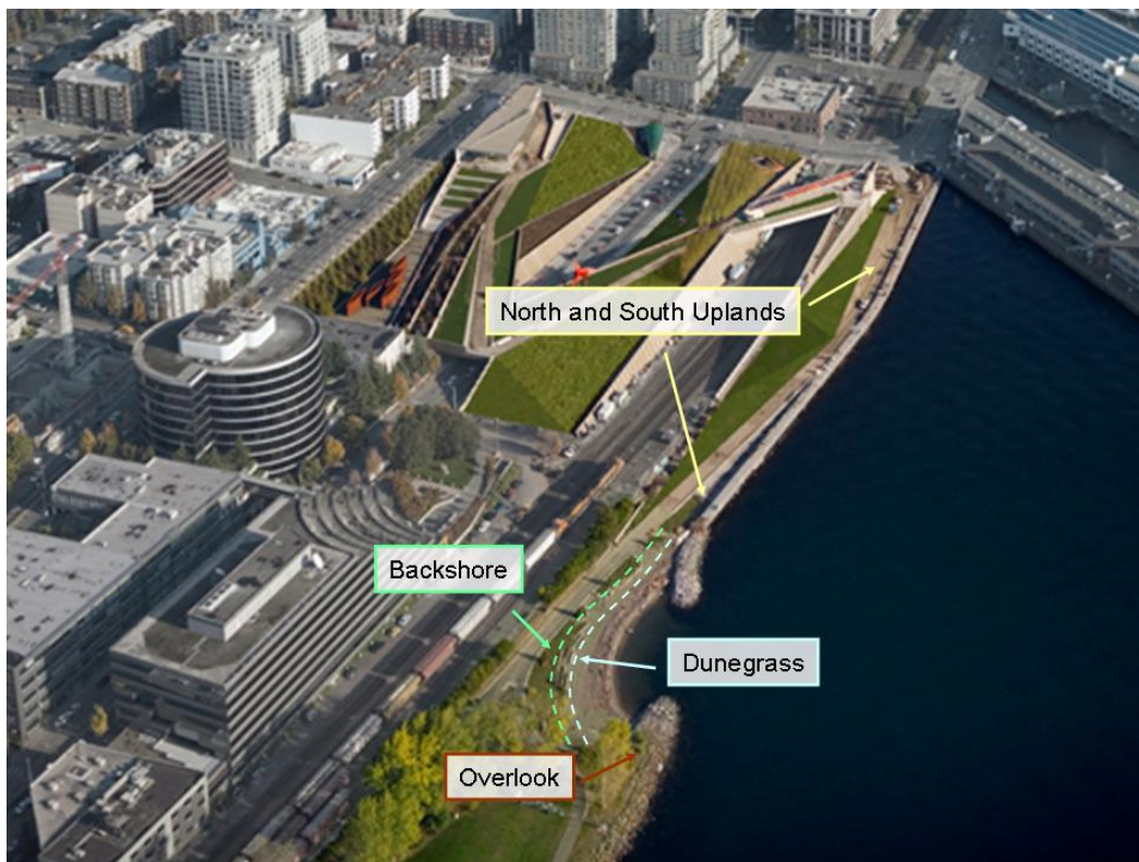
Figure 5. Aerial view of the Olympic Sculpture Park site after construction, showing vegetation sampling locations.
