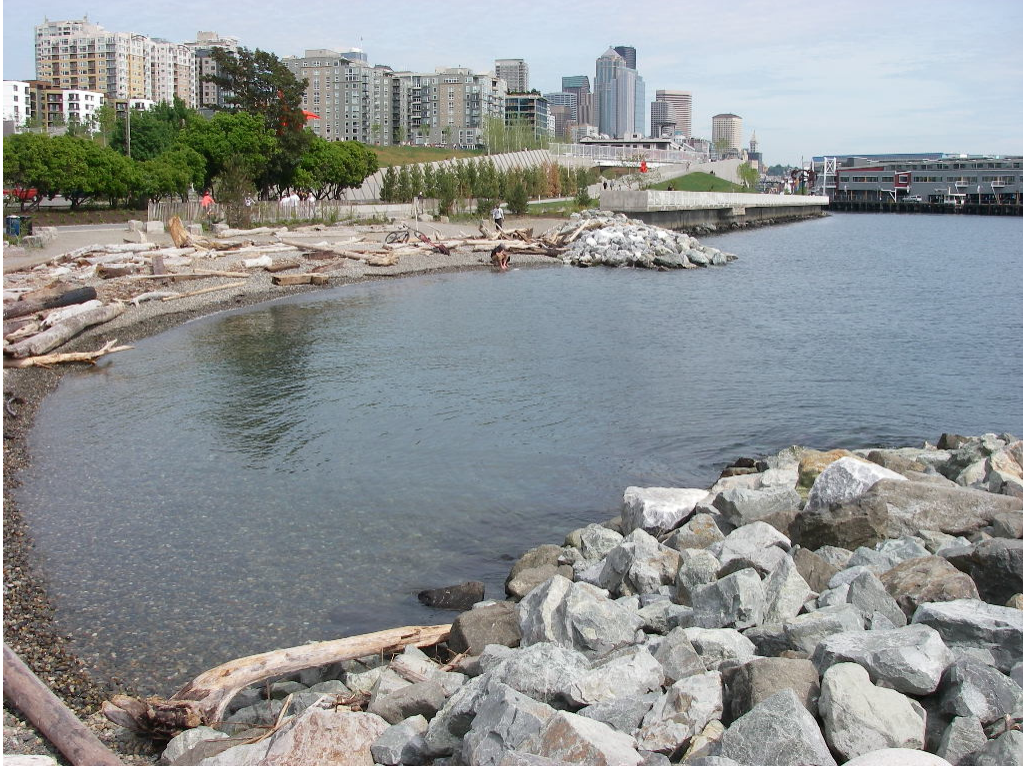
Figure 2. Photograph of the Olympic Sculpture Park site after construction at high tide, showing inundated pocket beach and habitat bench strata.
